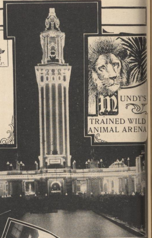
VIEW OF TOWER AT NIGHT
