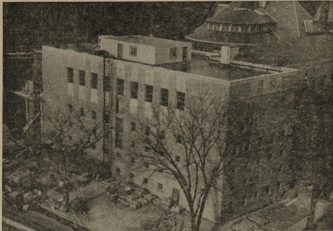
PROGRESS —Last year at this time the new law library, being built on Lathrop dr., was nothing but a conglomeration of orange steel beams. In this recent picture, progress on the building is shown. The beams are covered by a layer of rough red brick, and this layer is covered by a layer of smooth-finished cream-colored brick. Glass panes are in the windows, and the workmen are completing the inside of the library.
