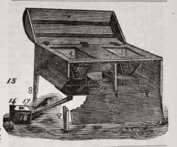
extracting, beekeepers must have a commodious storage for uncappings, so that they can drain thoroughly, leaving little or no honey to be put in the solar extractor. With this end in view, I made my uncapping table, and when completed, was thoroughly satisfied with it, at least, for my own use.
