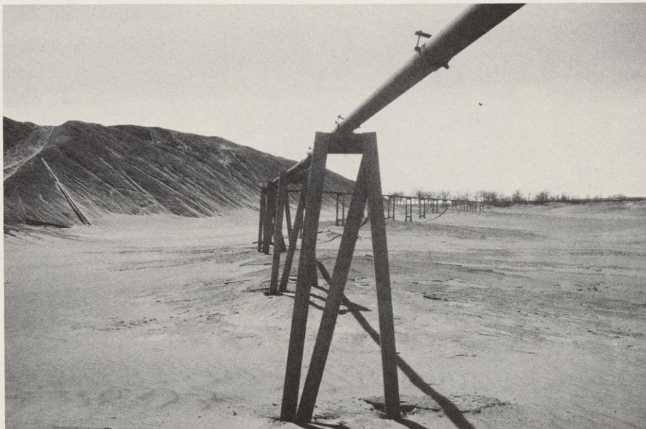
This discharge pipe once carried slurried wastes from Eagle-Picher's Schullsberg zinc and lead mine. The mine is closed now, but pollutants from the flooded shaft contaminate area wells.
