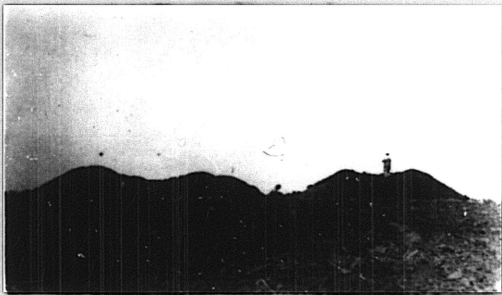
Heaps of Earth thrown out in Excavating H.S.X-10. From south.
