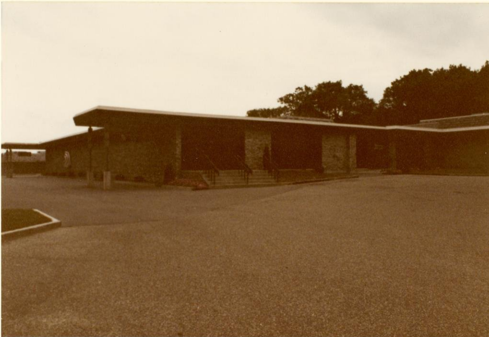
Entrance to Restaurant Wing - Includes the Scandinavian Room
