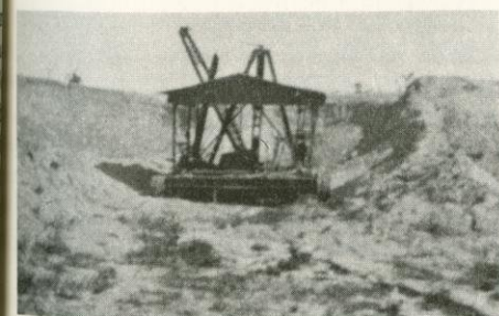
The electric shovel mentioned in the monograph about Brickmaking. Notice how clumsy and unwieldy it is. The ramp to the left was for the "tram" which was pulled by the "electric donkey." About 1928.
