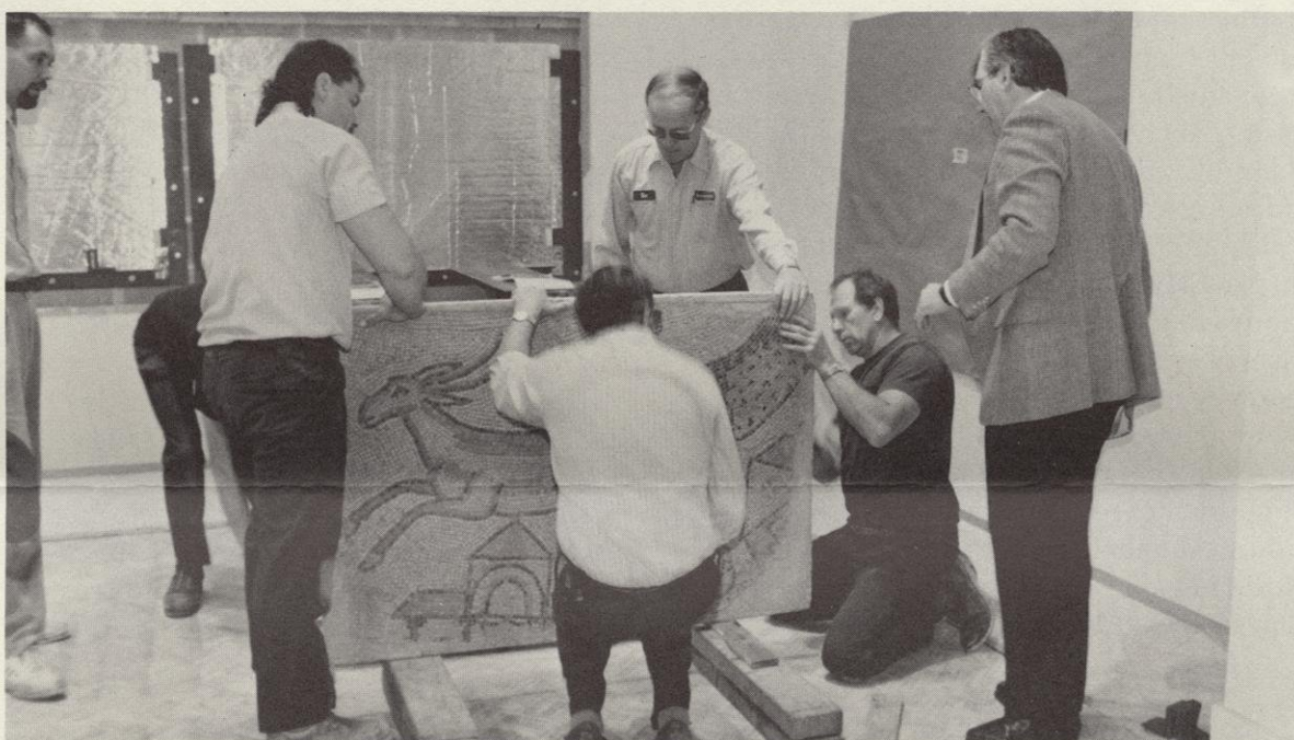
Once in the vertical position, the mosaic must be moved into place in the wall. Finally the mosaic is bolted in place supported by steel on three sides and flush with the wall surface. University engineers determined that the mosaics are actually safer when stored vertically rather than horizontally, for the stress is more evenly spread out.
