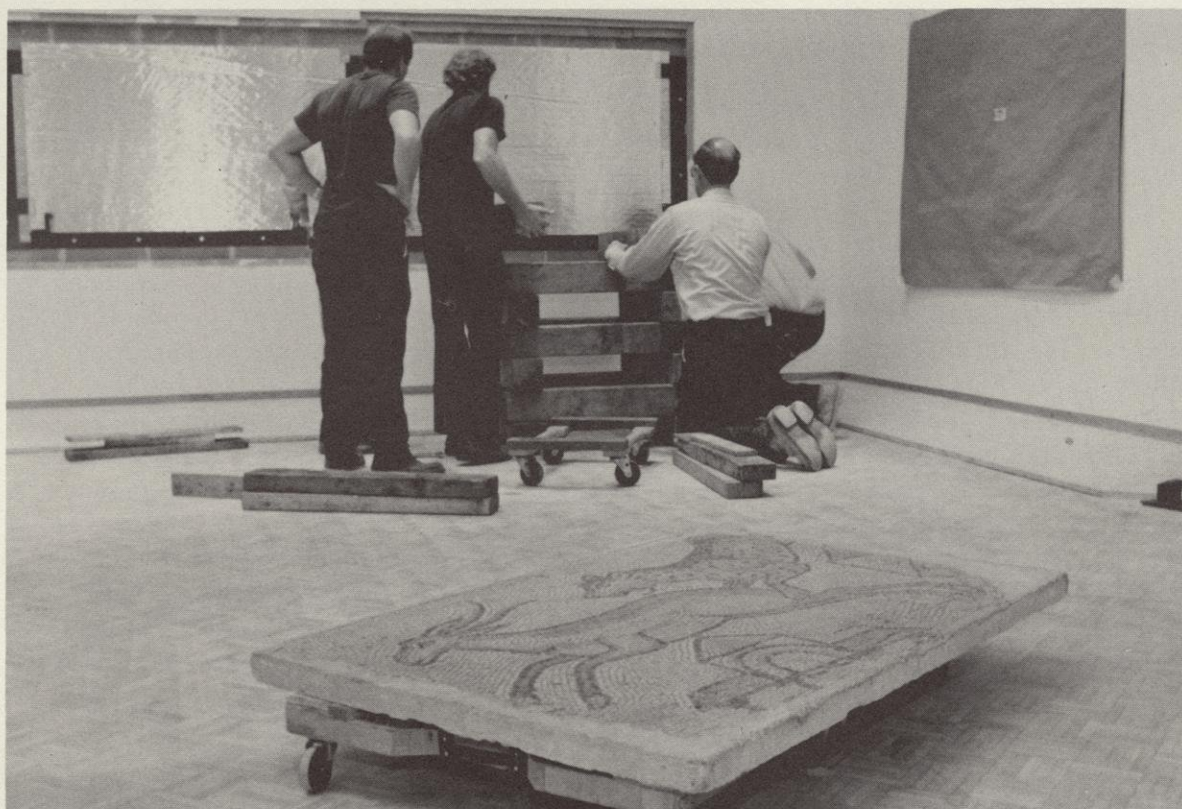
Special cuts have been made in the wall with steel brackets to accommodate each mosaic. The first task is to move from horizontal to vertical position without changing the stress; next the work must be raised to installation level.
