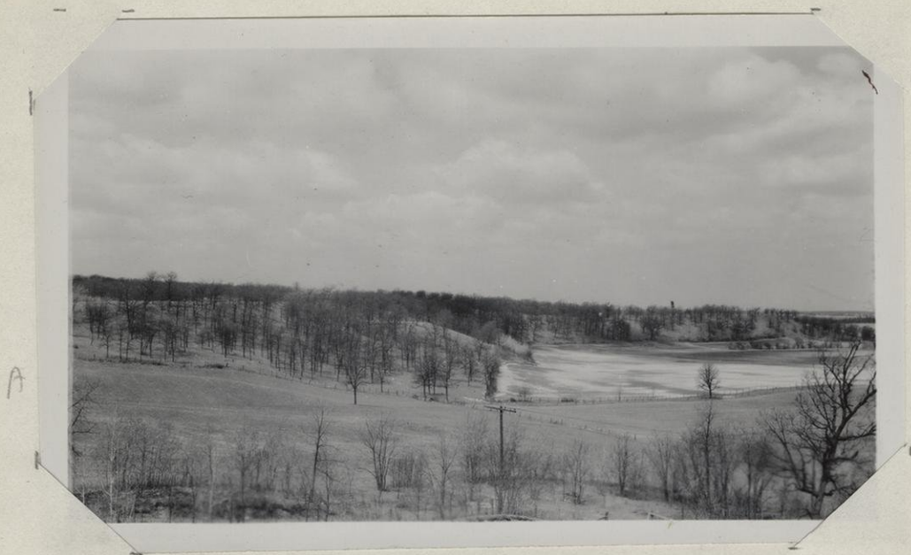
336 Drainage channel east of Delafield.
