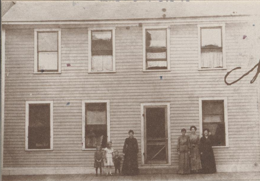
The boarding house was home for single men working at the mill in the early days. This view is the kitchen side.
