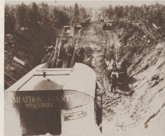
Building the road up Brokaw Hill.
