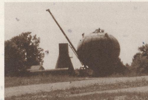
The new water tower under construction.
