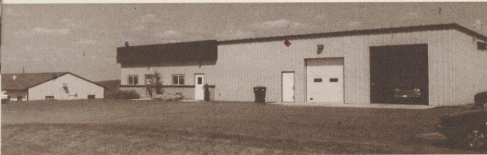
The Northside Business Park, operating in the new addition to Brokaw.
