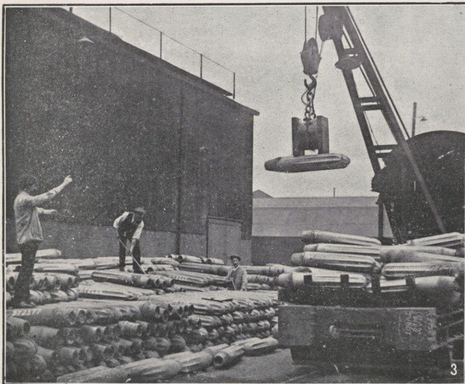
1. A Heap of Raw Material for making High Explosive Shell Steel. 2. Tapping a Charge from an Open-hearth Furnace.
