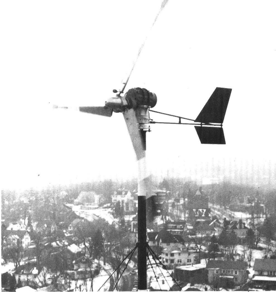
The ECE department wind energy conversion station harnesses wind power and supplements the local AC electrical system.
