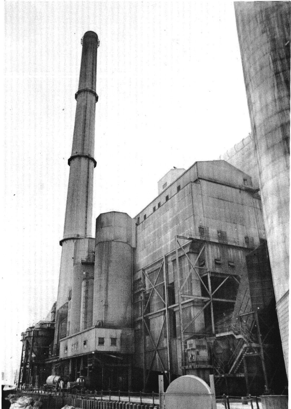
The Oak Creek Nuclear Power Plant, Wisconsin
