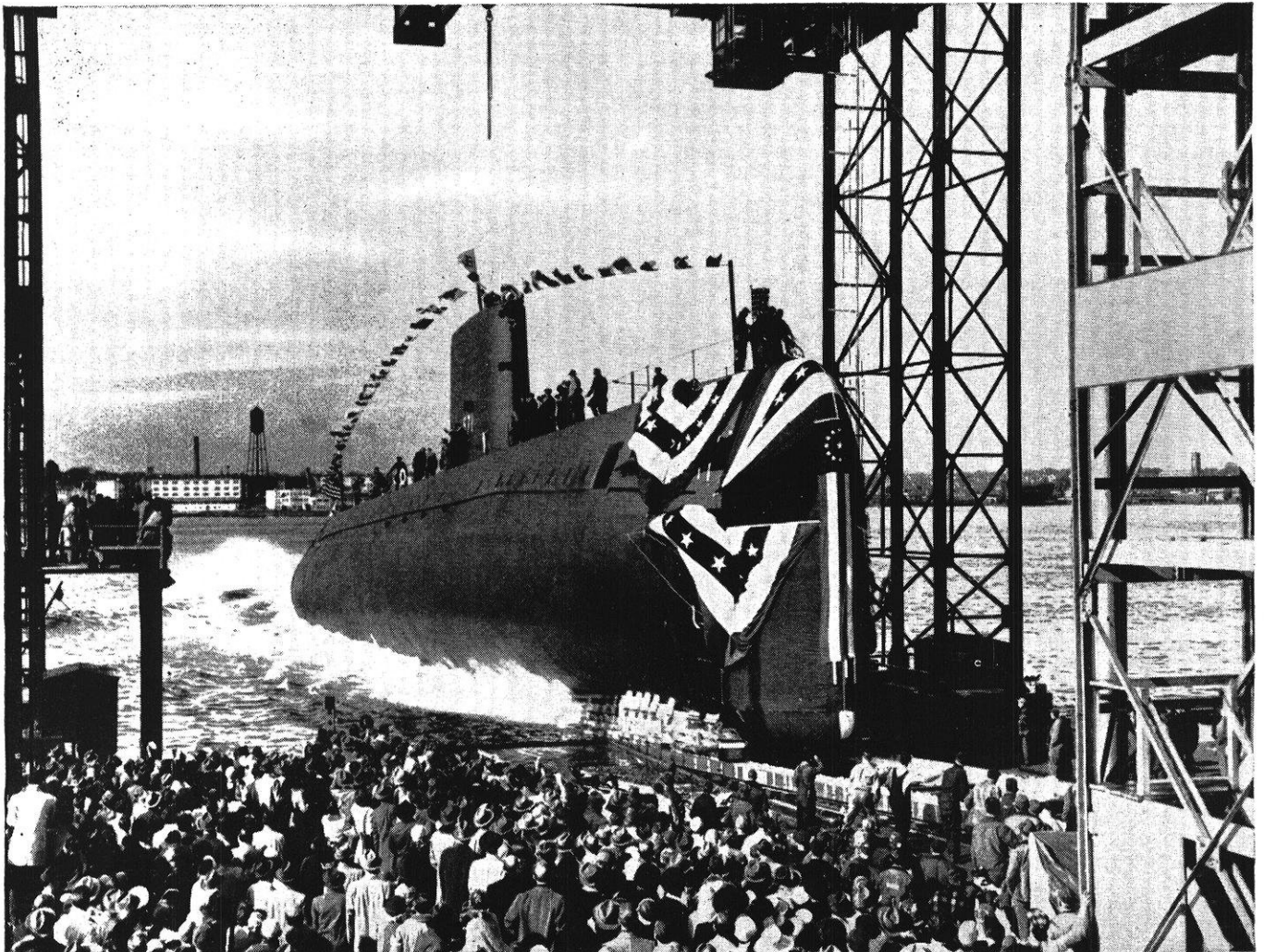
SLIDING DOWN THE WAYS at Groton, Conn., goes the USS Nautilus, newest and fastest member of our undersea fleet. During welding, Worthington heavy-duty turning rolls rotated the hull sections.
