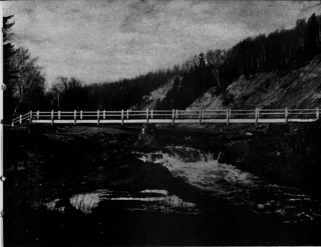
New bridge across the Bad river, Copper Falls State Park.
