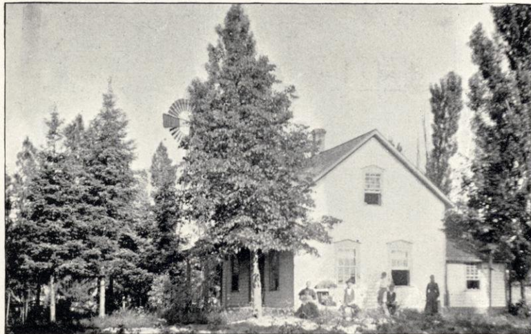
Residence of Mr. Fred Pipgrass of Green Valley, near Pulcifer.
