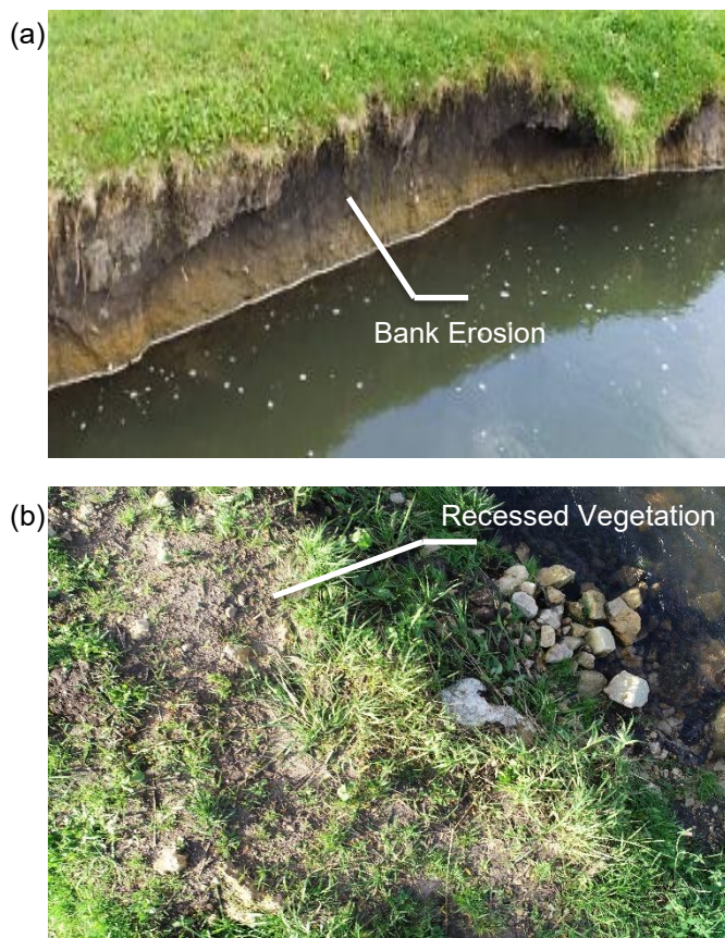
Figure 1-2 | Flood-induced stream habitat health losses in Black Earth Creek. (a) shows the bank erosion with bare soil after the August-2018 flood event; (b) displays the riparian vegetation recession and exposed stream bank after the same flood event.
