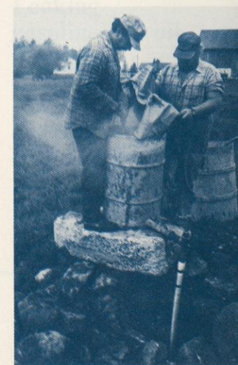
Well workers mix a cement grout to pour down and seal an abandoned drainage well.
