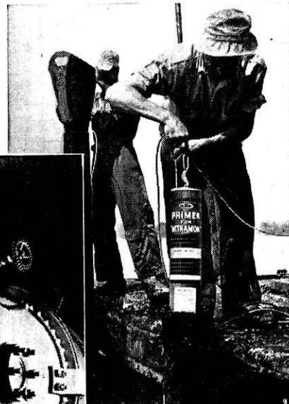
A. L. St. Peter, Princeton '37, supervisor blasting operation Susquehanna River Project, lowers a 5½ inch "Nitramon" Primer into one of 600 drill holes preparatory to blasting a pipe line ditch.
