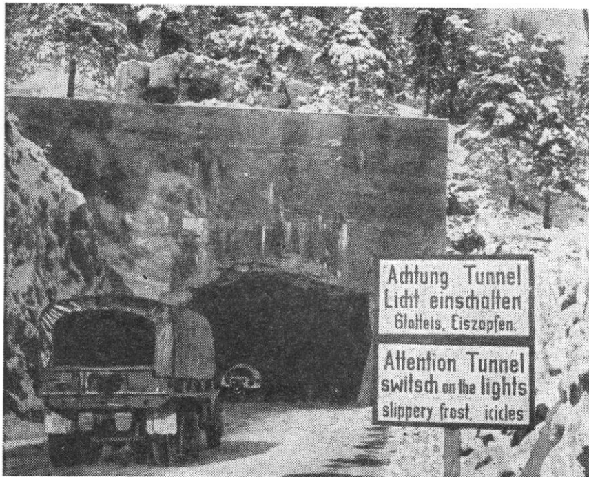
The double tunnel at Eschenlohe, on the main road between Munich and Garmisch, has been reopened. During the war it served as an underground Messerschmitt plane factory. Heavy charges of dynamite were used to clear the tunnel for the resumption of traffic. (DENA-Bild)
