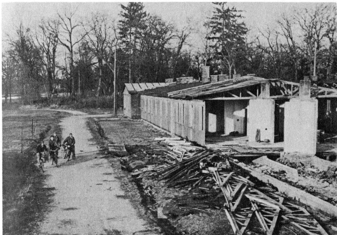
The Biederstein Youth Center in construction
