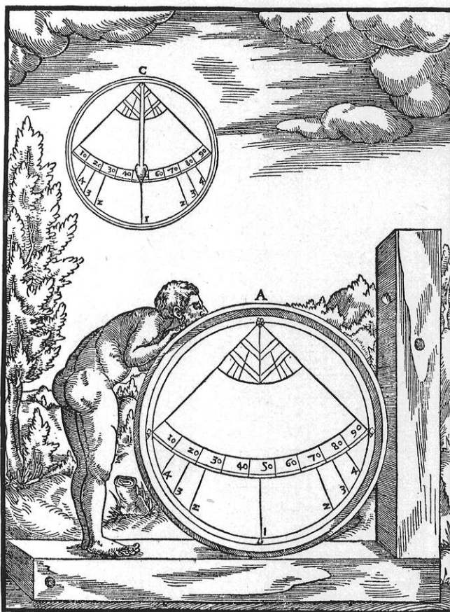
An ancient Roman surveying level from Herbert Hoover's Translation of Agricola
