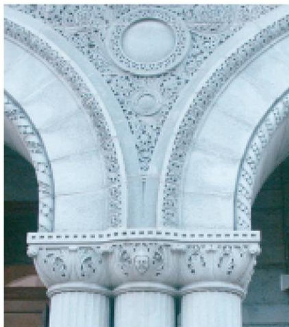
Architectural detail, Milwaukee Federal Courthouse. (Kathleen Sitter, LRB)
