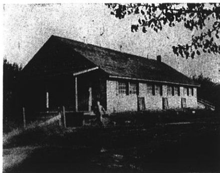
Packing room above, with storage below. The air intakes to the basement (where the shutters are lifted) are sufficiently large. The small outlet flues in the crown of the roof are entirely inadequate.
