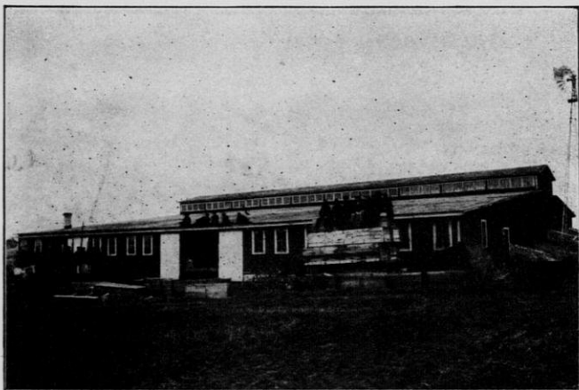
Nursery packing shed and storage cellars.
