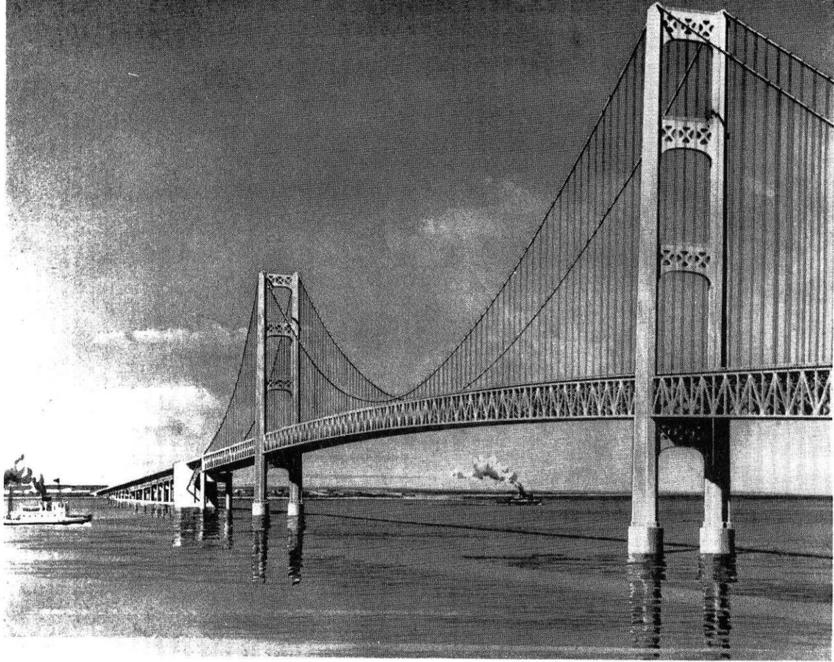
Fig. 1.—Two main steel towers rise majestically 552 feet above water from piers founded on rock approximately 195 feet below lake level. These main towers support cables for a center span of 3800 feet, second only to the 4200 feet of the Golden Gate Bridge in San Francisco. The total length of the bridge and approaches is 26,195 feet, while the suspension bridge, 8,614 feet from anchorage to anchorage, is the longest in the world.
