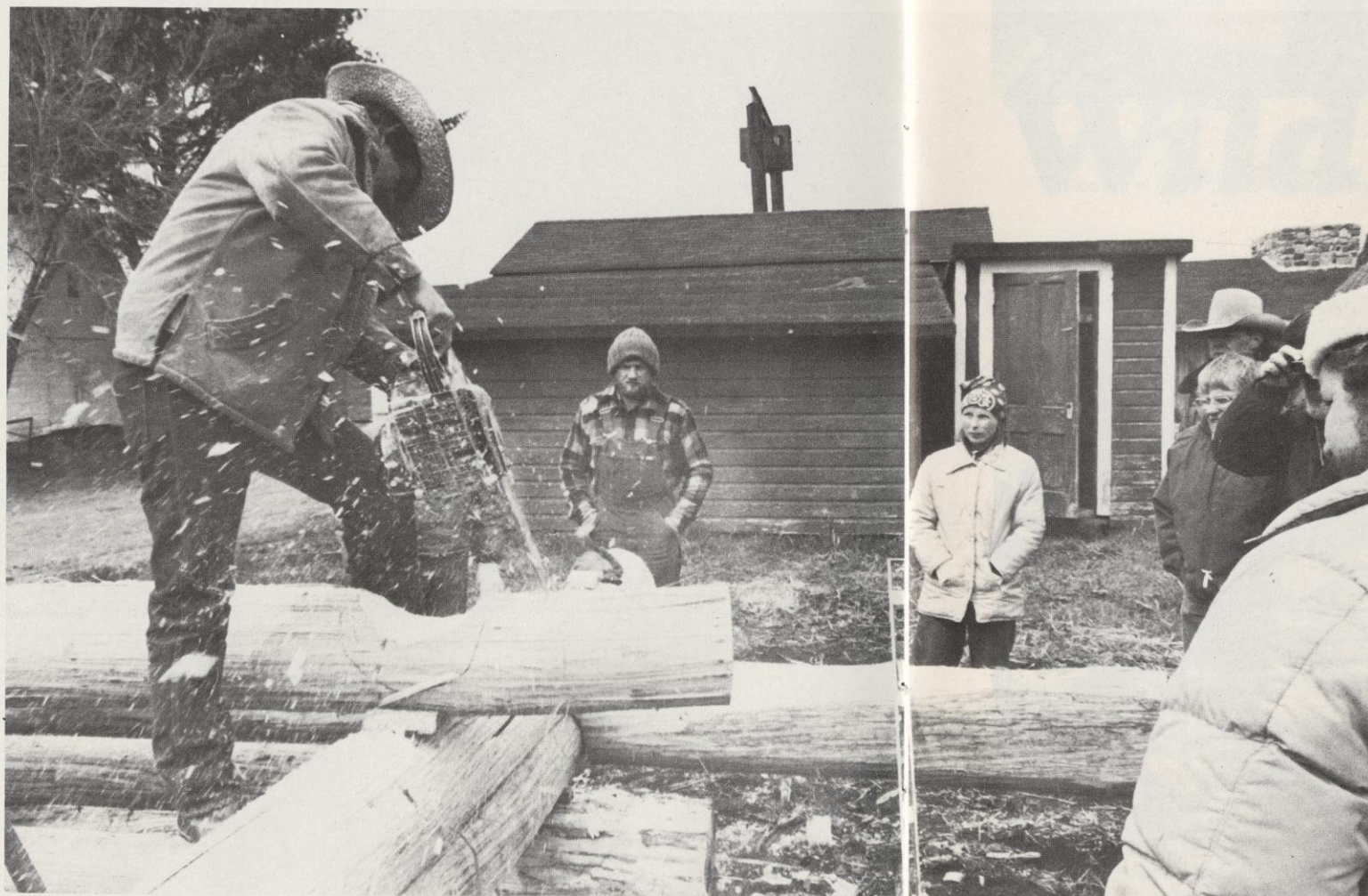
Palmquist demonstrates scoring a notch with a chain saw. Photo by Cedric Vig
