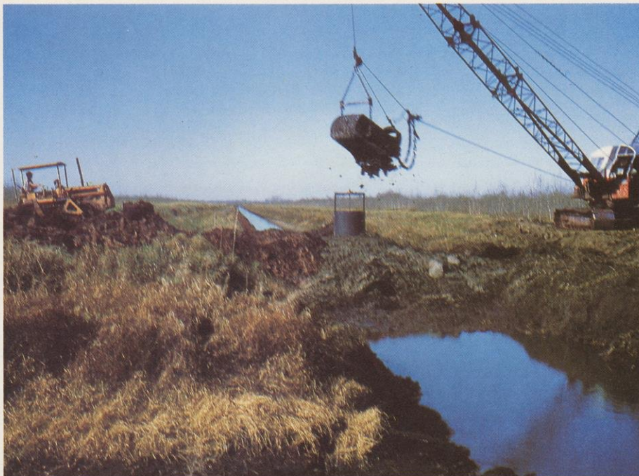
Dragline constructs flowage channel to improve wildlife habitat at Mead.
