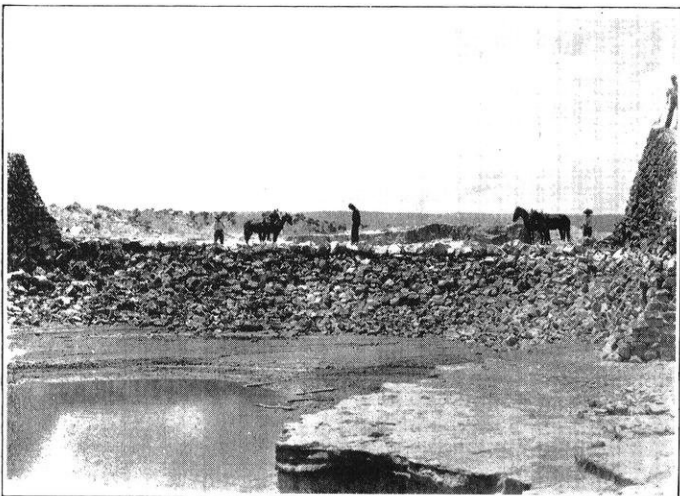
FIG. 2 — Spillway of an earth dam.
