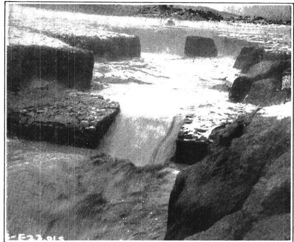
FIG. 1 — Checkdam in flood.
