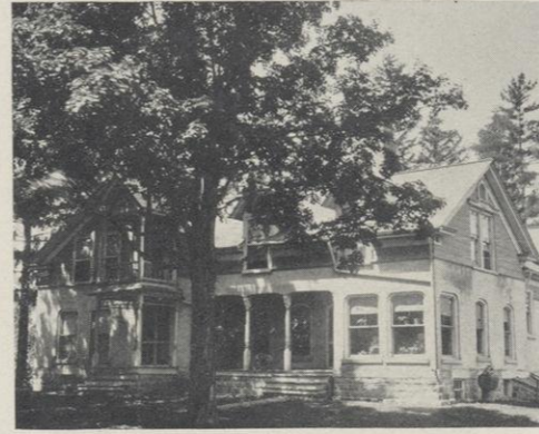
RESIDENCE OF W. E. HOYT Rochester Township
