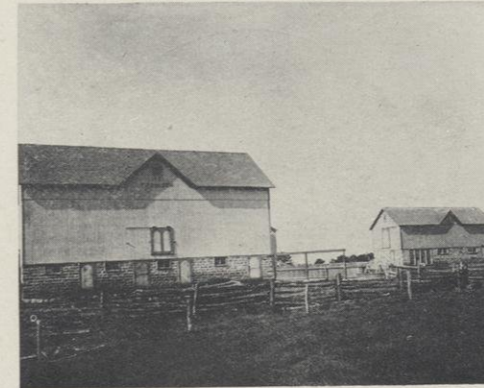
FARM BUILDINGS OF THOMAS PAULSEN Rochester Township
