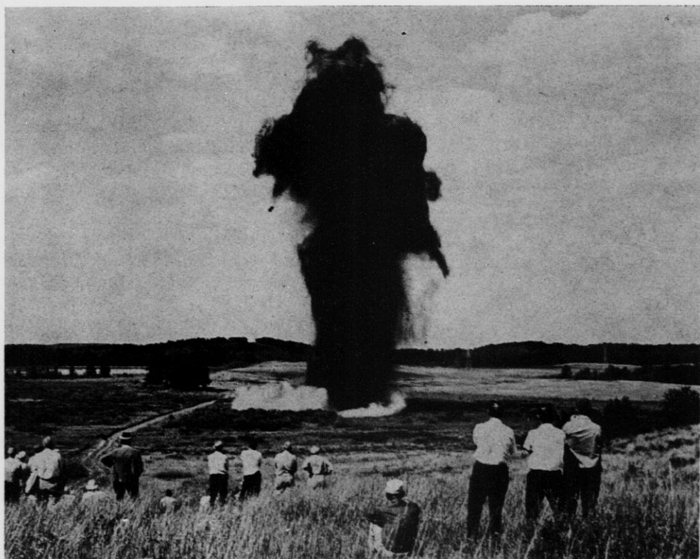
Public interest runs high regarding pothole blasting to develop wildlife habitat. Research broke the cost barrier by adapting ammonium nitrate (a common fertilizer) and fuel oil to serve as the explosive. About $3 pays for a blast such as this.
