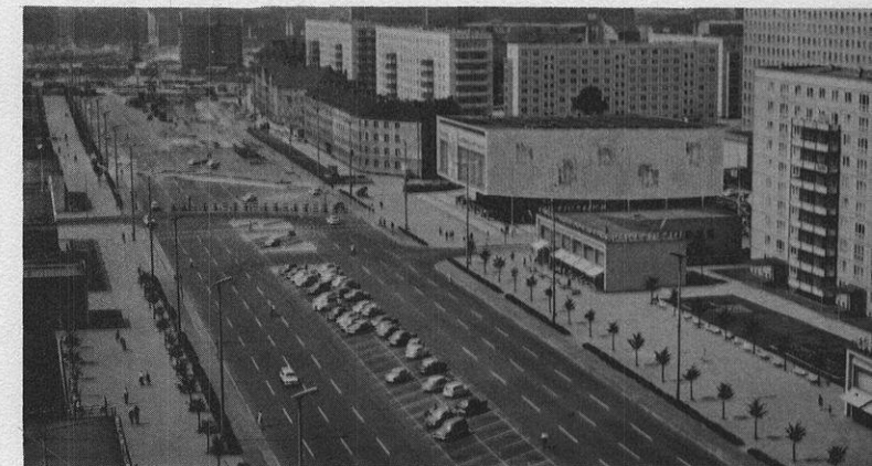
View from the top of the Haus des Kindes down the Karl Marx Allee toward the reconstruction of the Alexander Platz in East Berlin.
