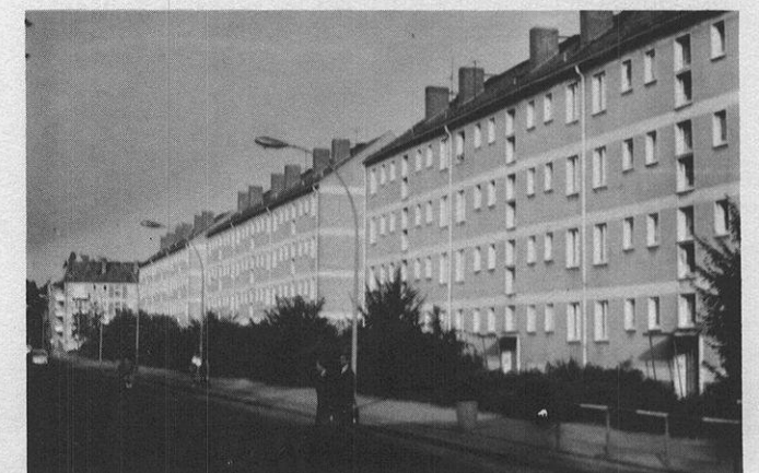
Uninspiring post-war apartment dwellings in Potsdam. Much of this city of several hundred thousand people remains untouched by the modern turn in East Berlin.
