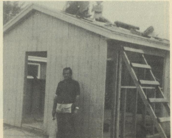
Building a Cabin at Camp Blessing
