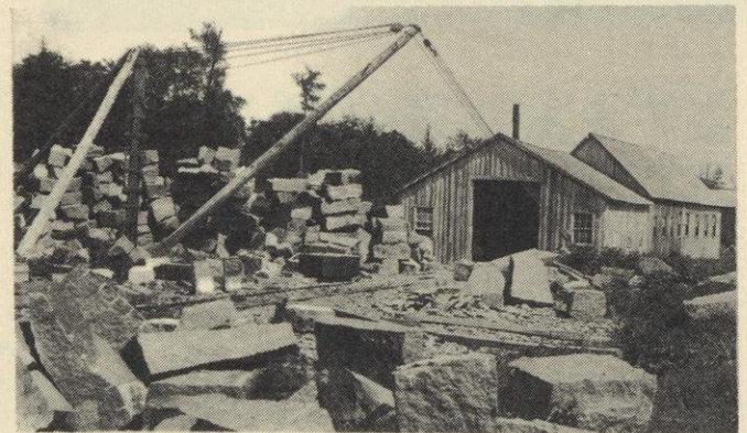
Manufacturing Shop at Upper Heights
