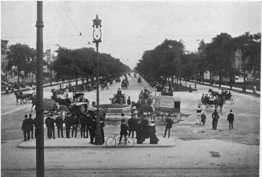
LOOKING SOUTH ON DREXEL BOULEVARD, CHICAGO.
