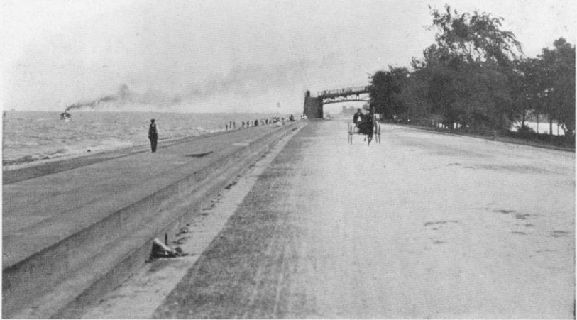
ON THE SEA-WALL, LINCOLN PARK.
