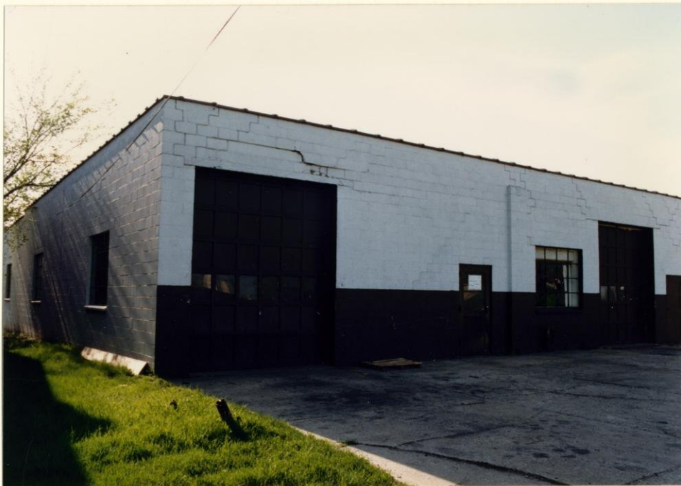
Beld Street entrance. Note cracks in exterior walls.
