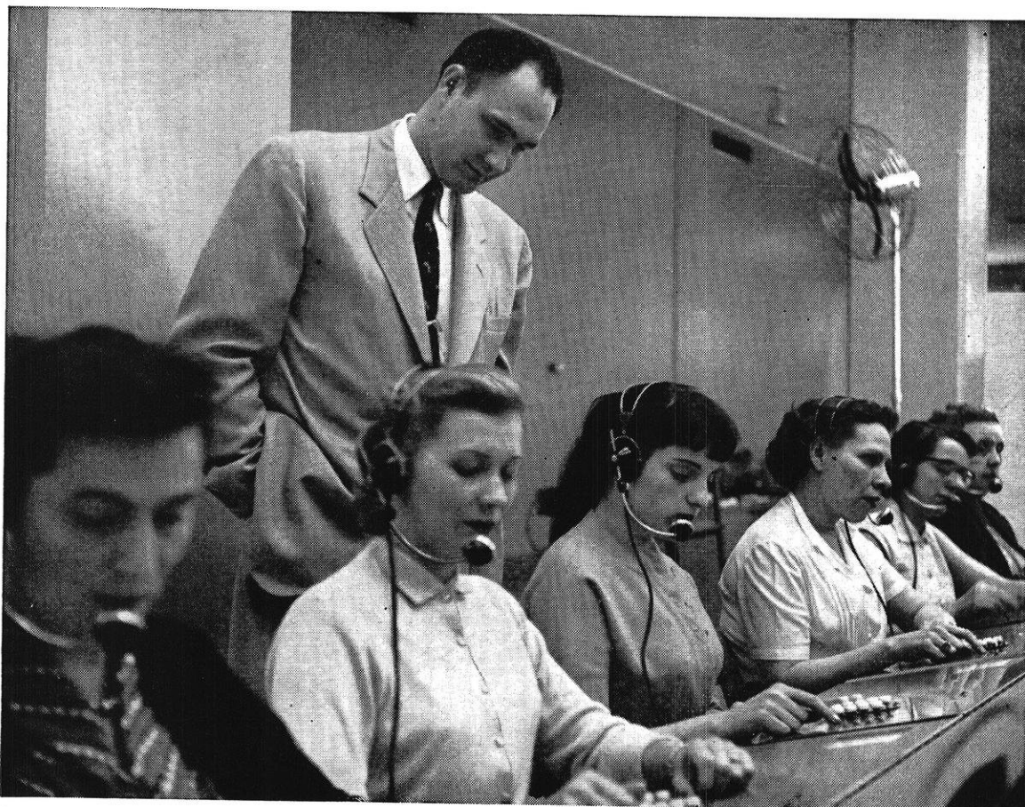
Emmett Smith, E.E., '50, supervises operation of the training switchboard which he originally helped to design.
