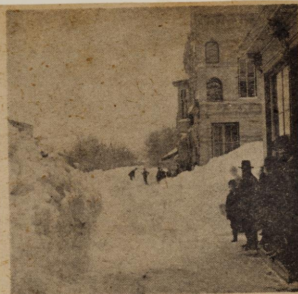
Taken from about 107 N. Ludington, looking south across James st. showing Griswold block on corner (Kroger Grocery) — Bay window second story is that in Dr. Poser's office above Kalks Drug Store. None of the people are identifiable, but prominent large man with hat could be John Sutton.
