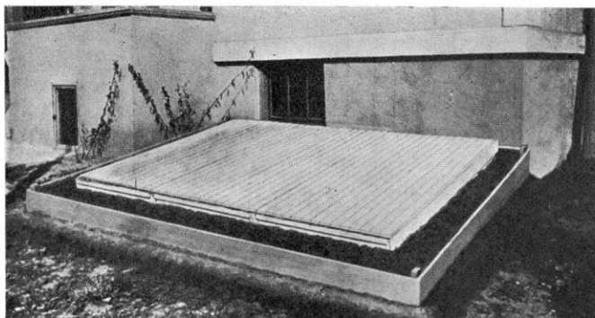
SAME FRAME ENCLOSED IN A SUBFRAME, THE MOATLIKE SPACE FILLED IN WITH LEAVES AND LITTER, AND THE GLASS COVERED WITH SHUTTERS FOR WINTER WARMTH.
