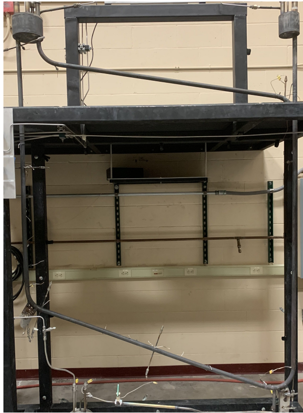
Figure C.12: Post-operation loop metal.
