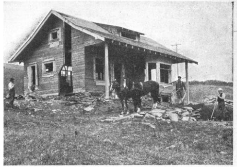
BUNGALOW IN PROCESS OF CONSTRUCTION.
