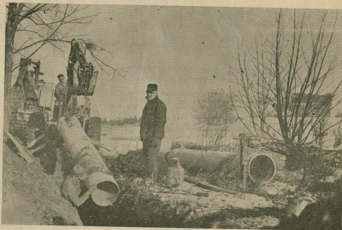
Brillion's interceptor sewer is well under way. Shown above as the Bahr Construction company crew getting a start with a light trench digger. Immediately beyond the tractor is the big trencher which is now in operation on higher ground. The view here looks toward the east immediately to the rear of the Earl Behnke property. (Staff Photo)
