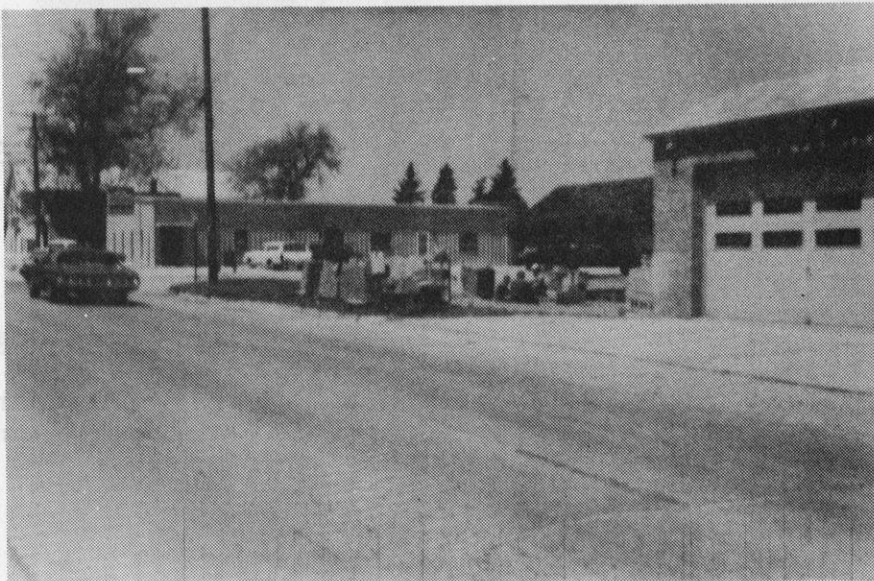
Pictured above is the Cleveland Fire Department. Construction of the new addition was begun in spring of 1976.
