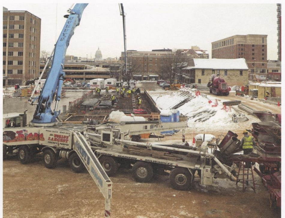
View of Chazen construction from the west, December 17, 2009. The Big Dog concrete pumper pours the floors on ground level. Photo: Russell Panczenko
