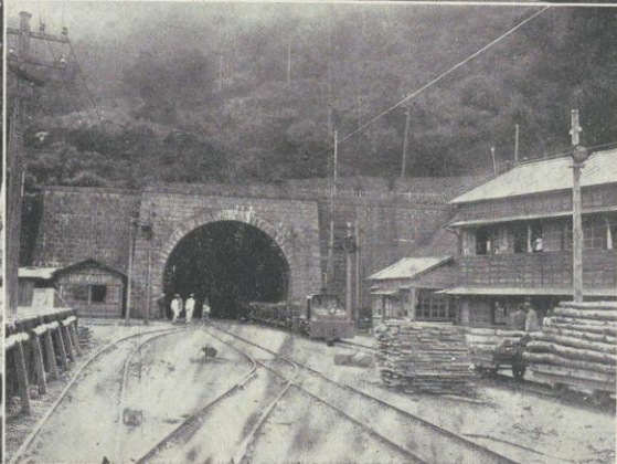
八、六、一八 丹那トンネルは着工以來十年の歳月を経て茲に見事開通す Tanna Tunnel bored through after ten years' continuous work. It saves hour's trip on Japan's main railway line. June 18.
