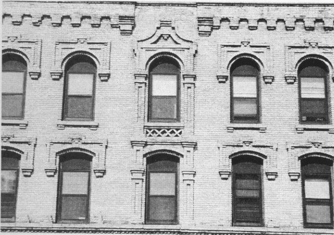
Fredendall Block (1868-1869), 33-39 S. Main St. George F. Schulze, architect.
