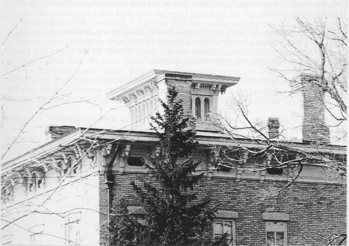
Timothy Jackman House (1858), 55 S. Atwood Avenue. Carefully crafted details, such as acorn pendants, adorn the cornice and lantern of this fine residence. The architect and builder have not been identified.
