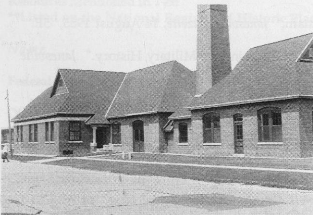
Janesville Pumping Station (1888). Photograph 1998.
