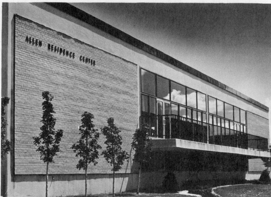
A new residence hall contrasts with early buildings.
