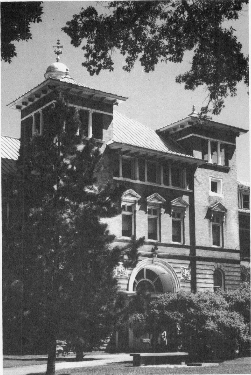
Old Main, completed in 1894, still stands although additions have been made to the original structure.
