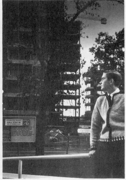
Construction of the first high-rise residence hall began in 1967.
