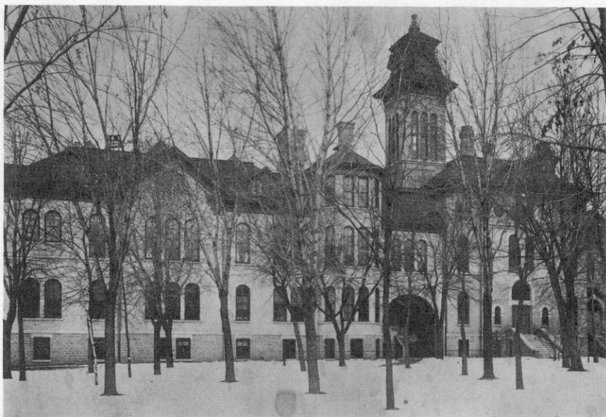
The original building of Oshkosh, completed in the summer of 1870.
