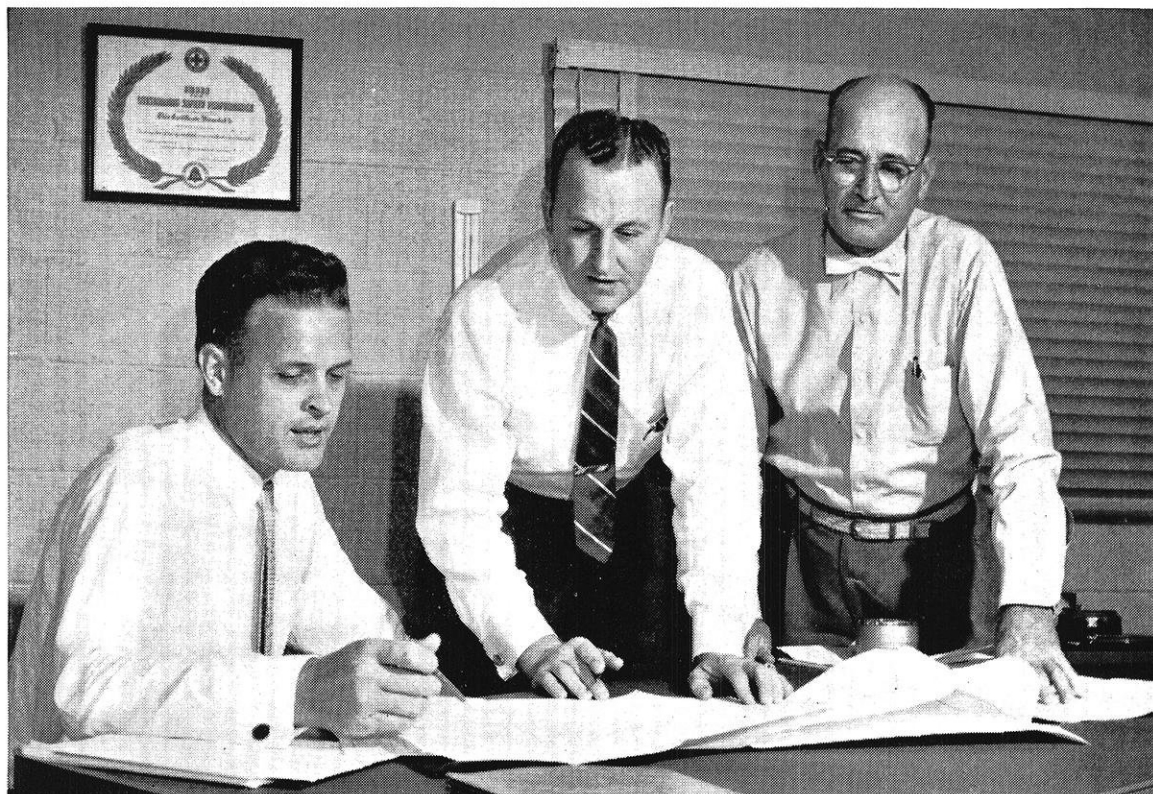
Planning for growth. Joe Hunt (left) talks with Jim Robinson (center), District Construction Foreman, and O. D. Frisbie, Supervising Repair Foreman. In Joe's district alone, 600 new telephones are put into service every month.
