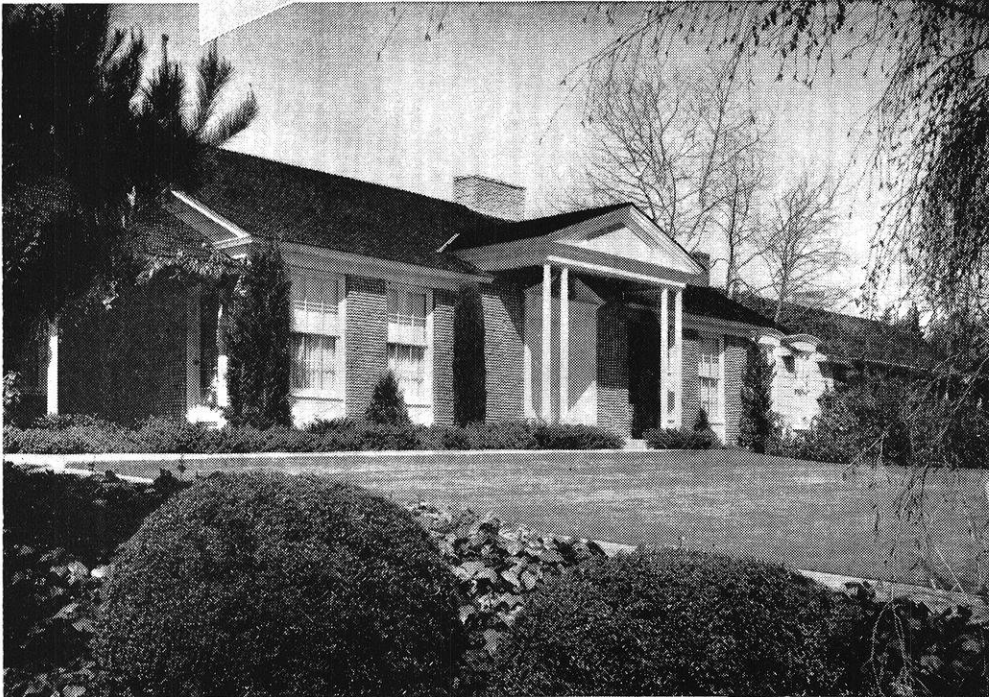
A Douglas engineer lives here
