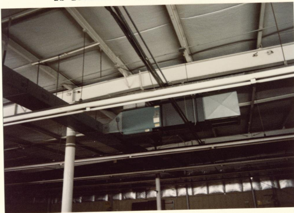
Exposed roof area of third addition contains suspended mechanicals. Note aluminum clad batt insulation on roof and walls.
