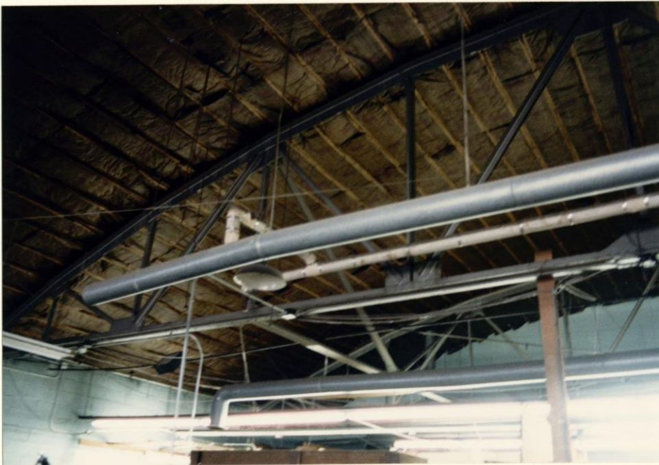
Barrel roof of original building. Note wood purlins and paper covered batt insulation. Roof is exposed in this back half of original building section.
