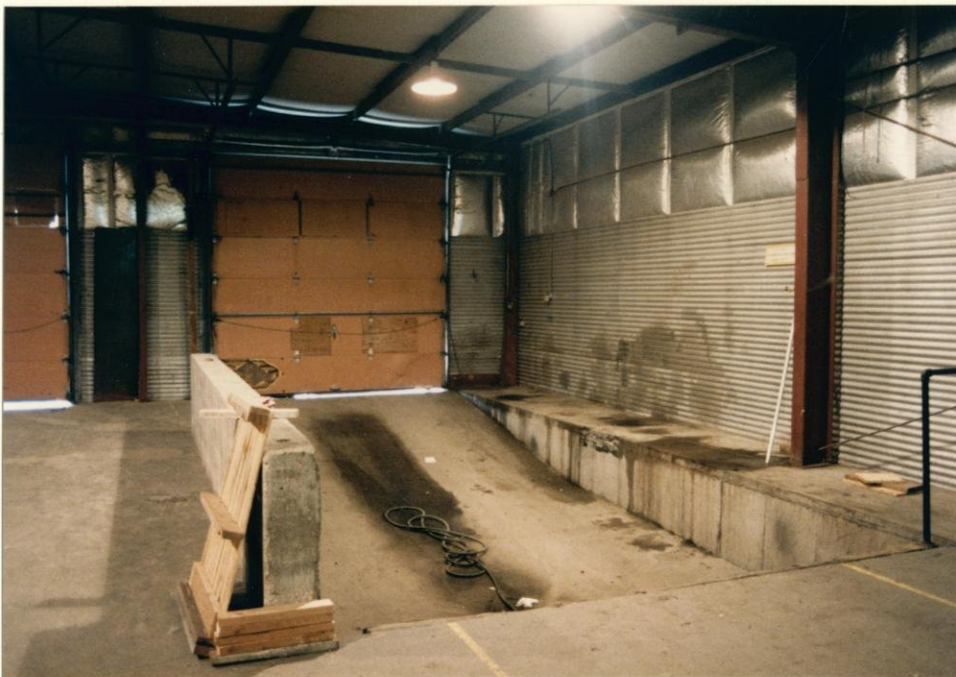
Interior view of truck dock located in third building addition; one ramp slopes to three feet below grade to create a truck height dock and the other entry is at grade.
