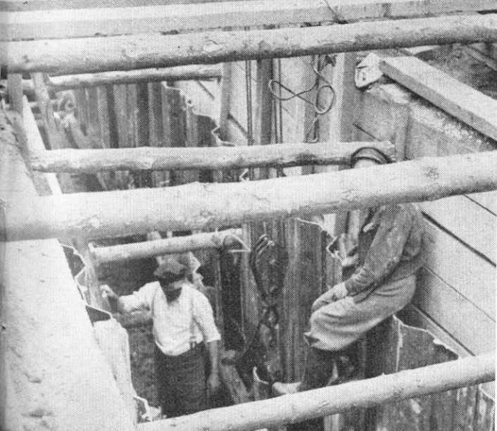
Steel pilings needed in soft soil of Luebeck add to costs.
