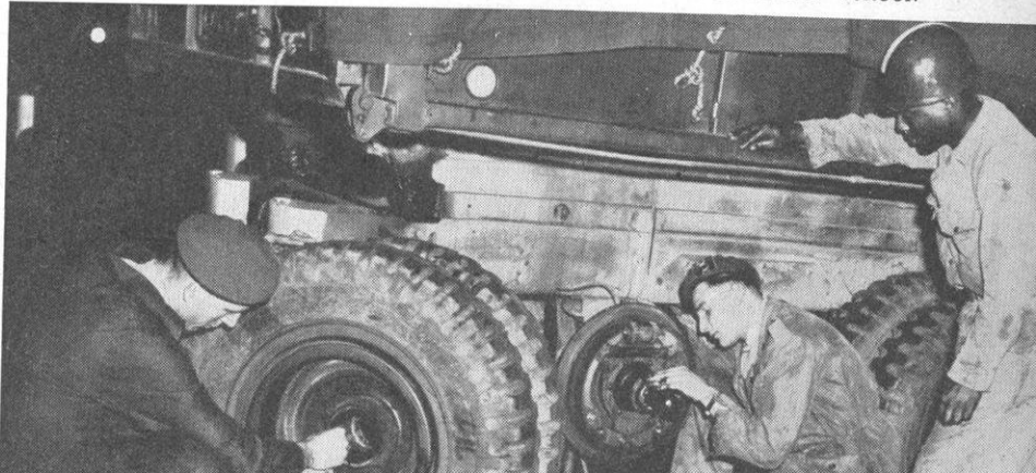
Pfc. Roger Winn instructs Dutch captain (cleaning brake drum) and sergeant-major (greasing spindle) in maintenance of 2 1/2-ton truck at MDAP school.
