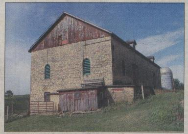
Photos courtesy Doug Cieslak, Driftless Area Land Conservancy The east-facing end of the barn shows tie bars that extend from the window louvers to the roof to make sure the roof won't sail away in a heavy wind.
