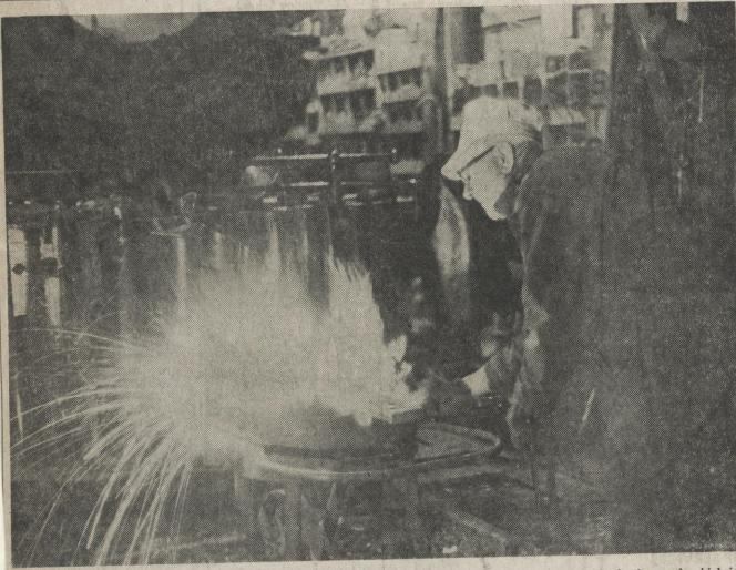
Rudolph Fluegel, 74-years-young, mans a glowing coal-fired forge at the repair shop of the Mid-Continent Railway Museum at North Freedom. He is working on repairs for the steam locomotive in the background, which is being restored for active service. (Stan Mailer Photo)
