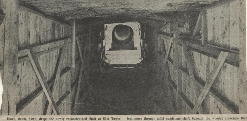
Down, down, down, drops the newly reconstructed shaft at Shot Tower Hill State Park near Spring Green. It was down this 80-foot drop plus 120 molten lead was dropped, cooling into balls as it fell.
