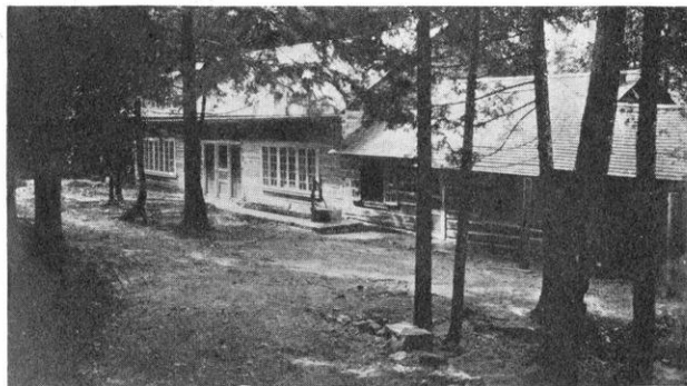
KITCHEN WING OF THE CAMP AFTER ITS COMPLETION.
