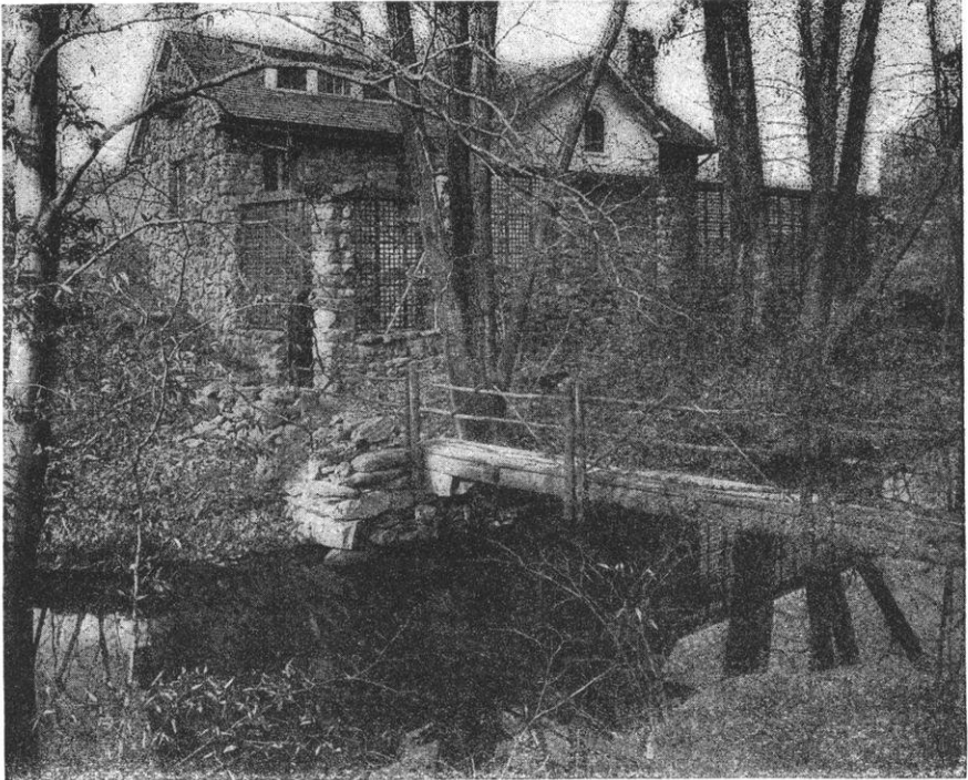
A SIMPLE RUSTIC BRIDGE ON THE HOOKER ESTATE THAT IS IN PERFECT HARMONY WITH ITS UNSPOILED WOODLAND SURROUNDINGS.
