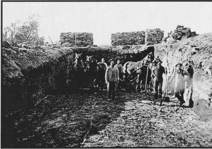
Digging the basement Circa 1861 or 1895
