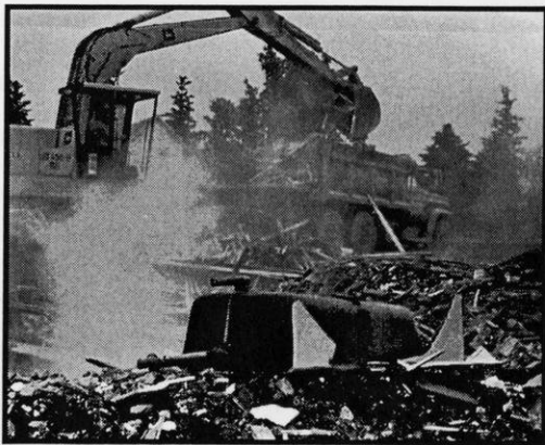
The demoliton of the " Gunderson Parsonage " in 1986
